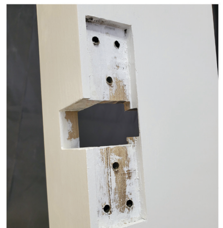
View of jamb face w/mortise cut out
