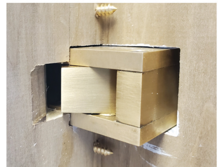
From inside jamb of hinge cut out
