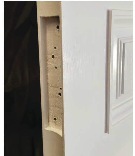
Door edge cut to 19/16" radius ready for hinge
